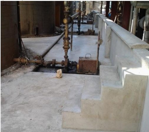
Tankfarm Concreting and Banding
